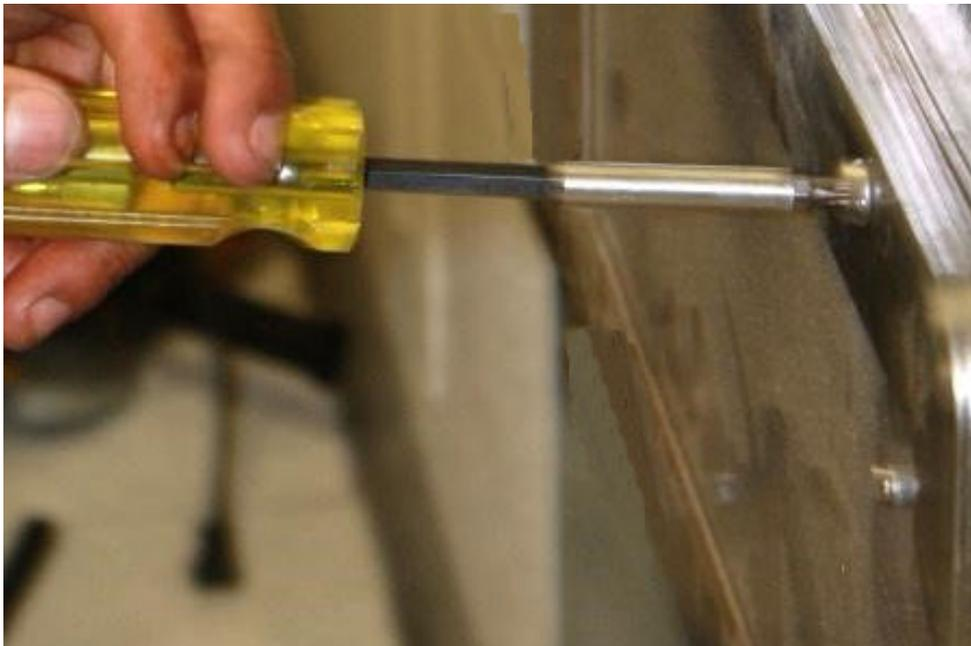
**Secure the PASS Frame to the cell door using the Security Screws supplied with your PASS unit. It is HIGHLY recommended that a screw thread adhesive such as “Loctite” or similar adhesive product be used on the threads of the Security Screws to assure a secure bond.**
