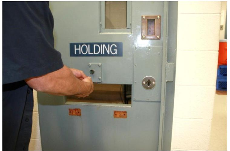
**After removing the cell's metal food slot door, locks and hardware, your cell door should look similar to the cell door below.**
