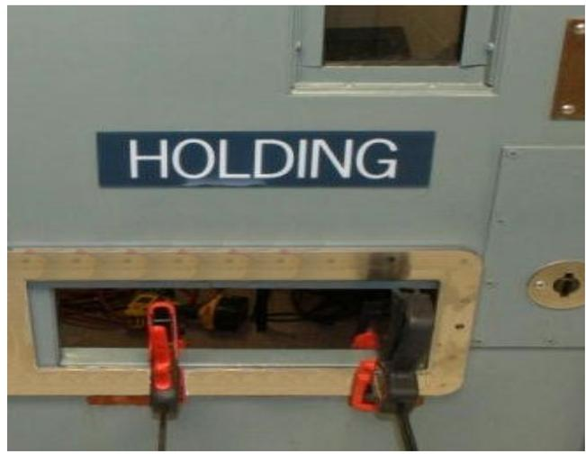
Next line up the PASS Door Frame to the cell door food port opening. Secure in place with clamps. **KEEP BOTTOMS OF FRAME & PORT FLUSH AND SMOOTH.**
