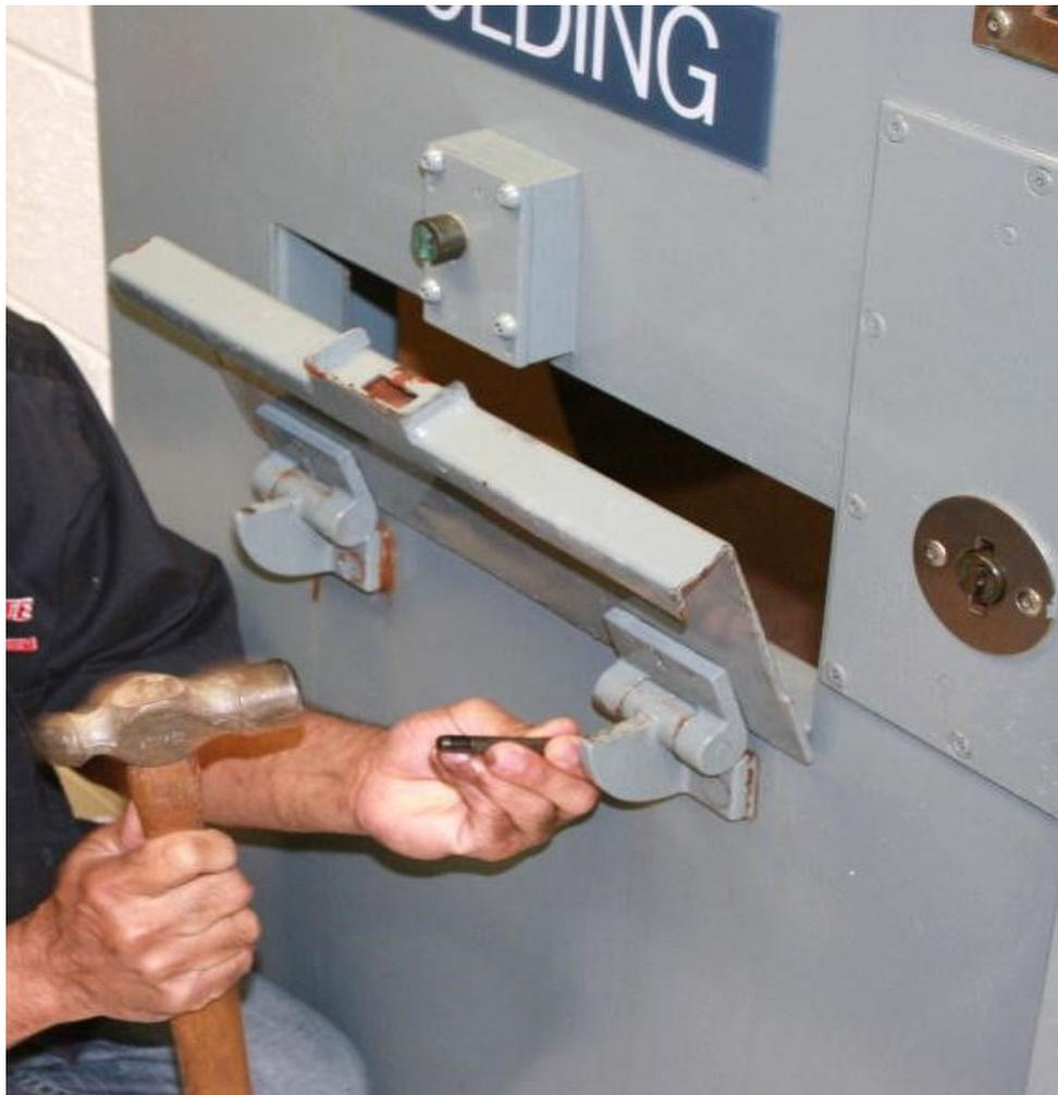
**First remove the metal door, the lock and all mounting hardware.**
