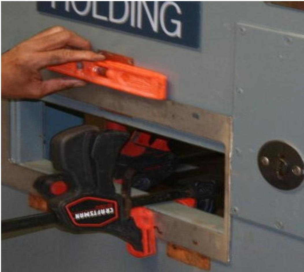
Make sure the bottom of the PASS Frame opening is level and in line with the bottom of the food port opening. Also make sure that both sides of the PASS Frame are evenly space with the sides of the food port opening.
