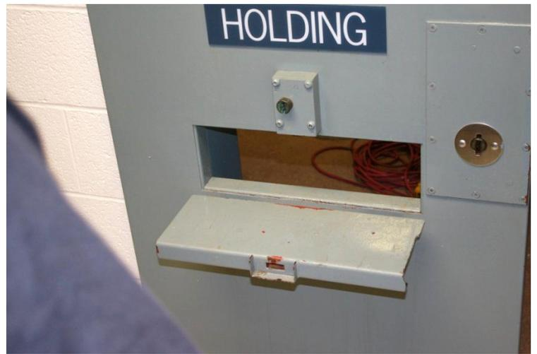
**Above is a typical cell door metal plate drop-down food door that will be replaced with the PATENTED ANTI-SPLASH SYSTEM (PASS) Frame.**
